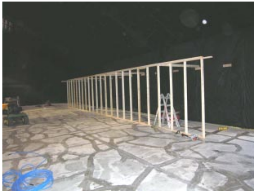
Looking East at end of work on September 16, 2006
