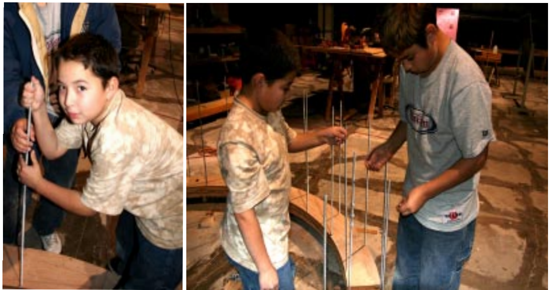
Angel (left) and Angel and Junior (right) insert support rods in the helix, add nuts and washers, and run them down the rods.
