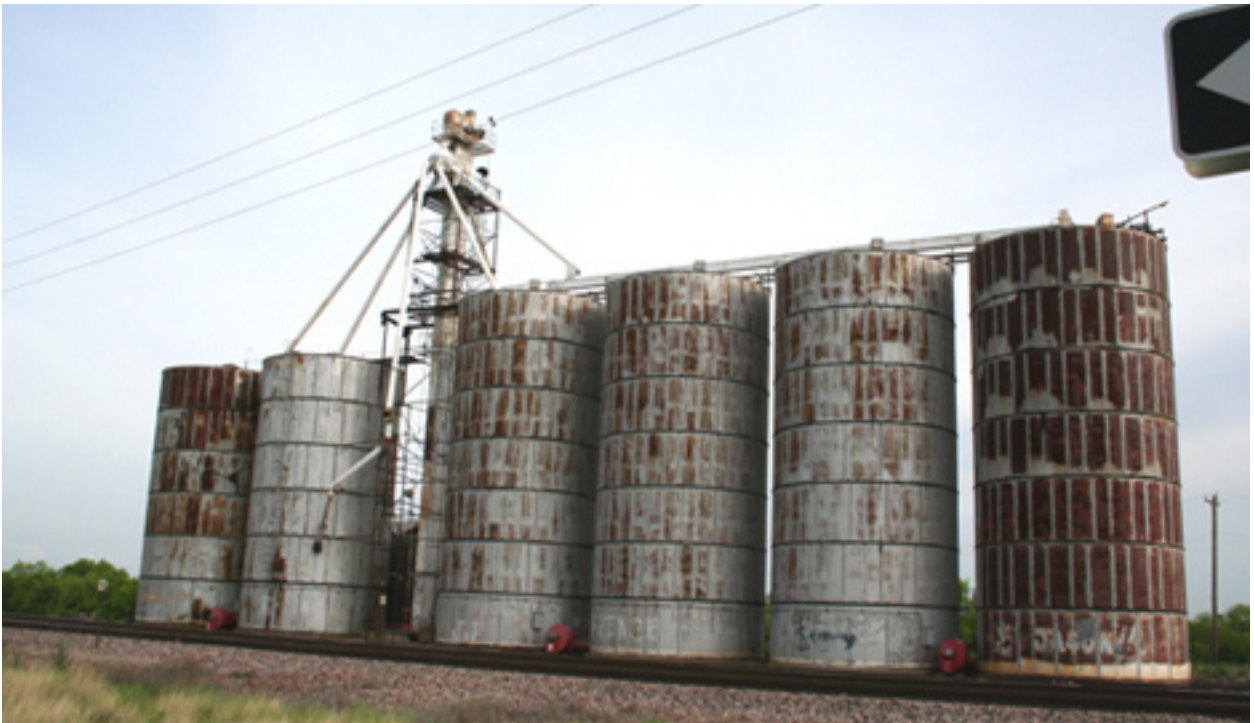
The North side of the elevator at Kirkland, TX. The bucket-type elevator mechanism is available from BH Models. The four tall tanks are about 56 feet high and about 24 feet in diameter
