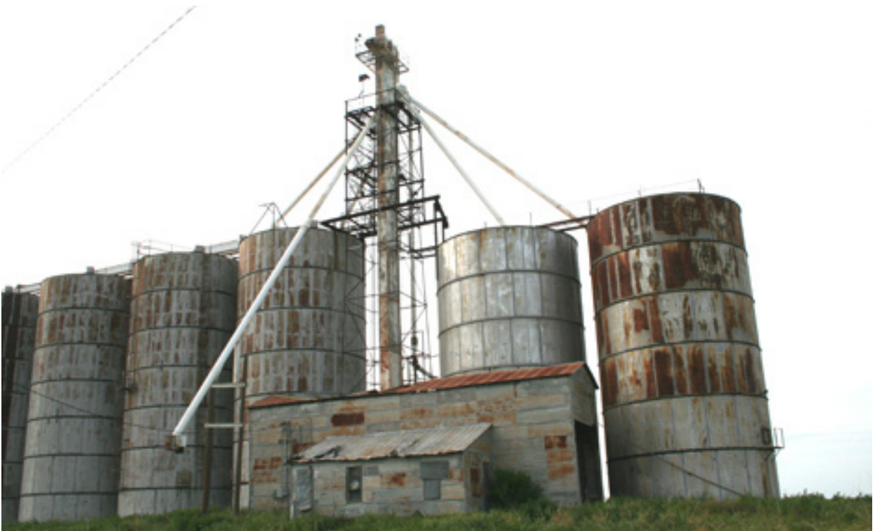
The South side of the elevator at Kirkland, TX. The dump house and office space are located here. The delivery pipe extending down this side is probably for truck loading. The dump house is about 20 feet to the ridge and about 45 to 50 feet long. Both photos dated May 7, 2007.
