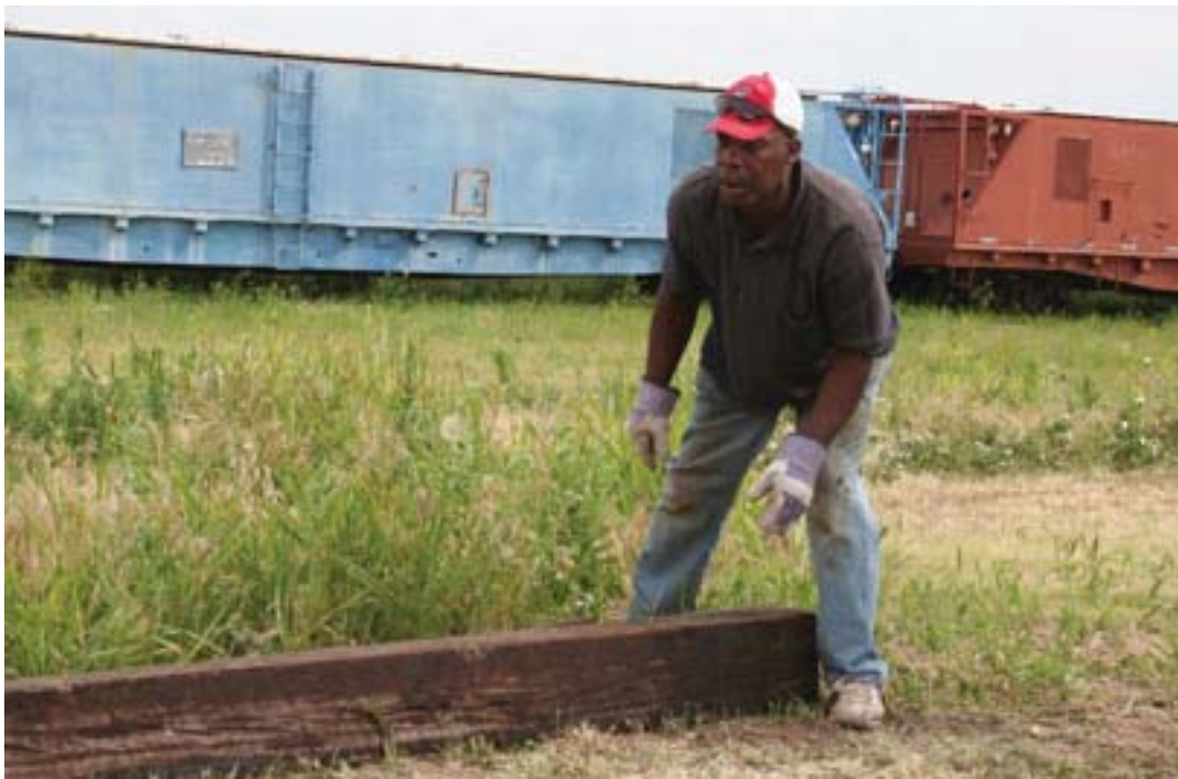
Roy ready to move a switch tie into position
