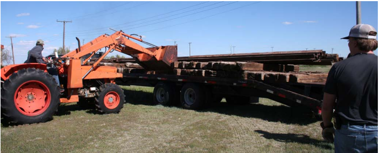
March 28, 2020: Initial attempt to unload materials at the Museum: Above: Tracy is using the loader to try to push the material off the trailer but this effort was unsuccessful. Below: In an attempt to unload the rail using brute force, Matthew Jusiak is on the trailer using a pry bar while Kenneth (foreground) and Chris pull on the ends of the rail. Meanwhile, Tracy went to fetch some other tools...
