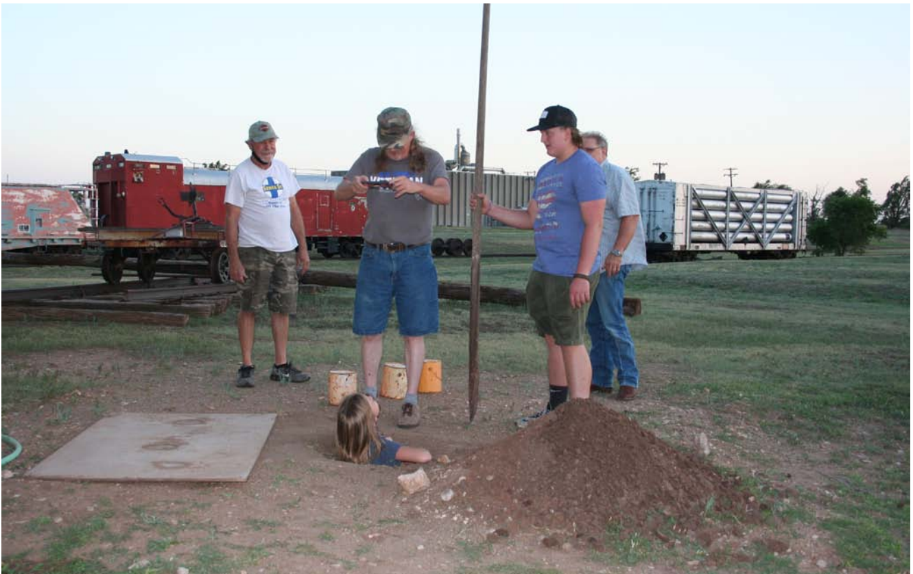
July 16, 2020: Above: Tracy is using a special long-handles shovel to remove loose dirt from the bottom of the hole for the utility pole while Kenneth, (David and Gail's granddaughter), Matthew and Chris look on. Below: Checking the depth of the hole. (She volunteered to get down in the hole!)
