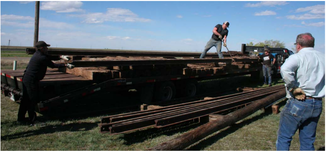
Above: The tools that Tracy fetched included a rail turner, rail tongs and tie tongs. This allowed the unloading to go much quicker with significantly less effort. Matthew is on the trailer rolling a rail toward the edge of the trailer while Bruce is attempting to help keep the near end straight, Chris is at the far end and Kenneth is standing out of the way.
