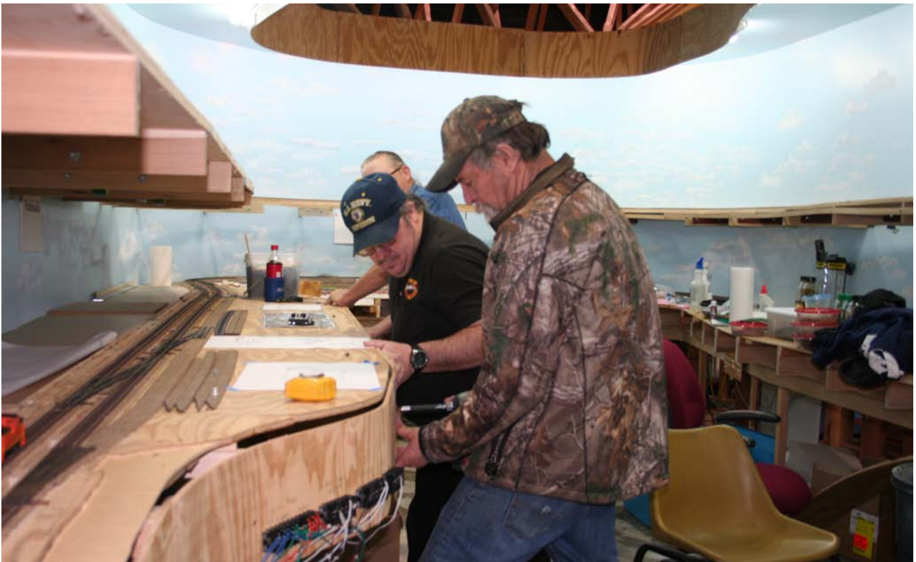
Jan. 25, 2020: Jimmy and Chris assisting Tracy in installation of plywood fascia around Panhandle.
