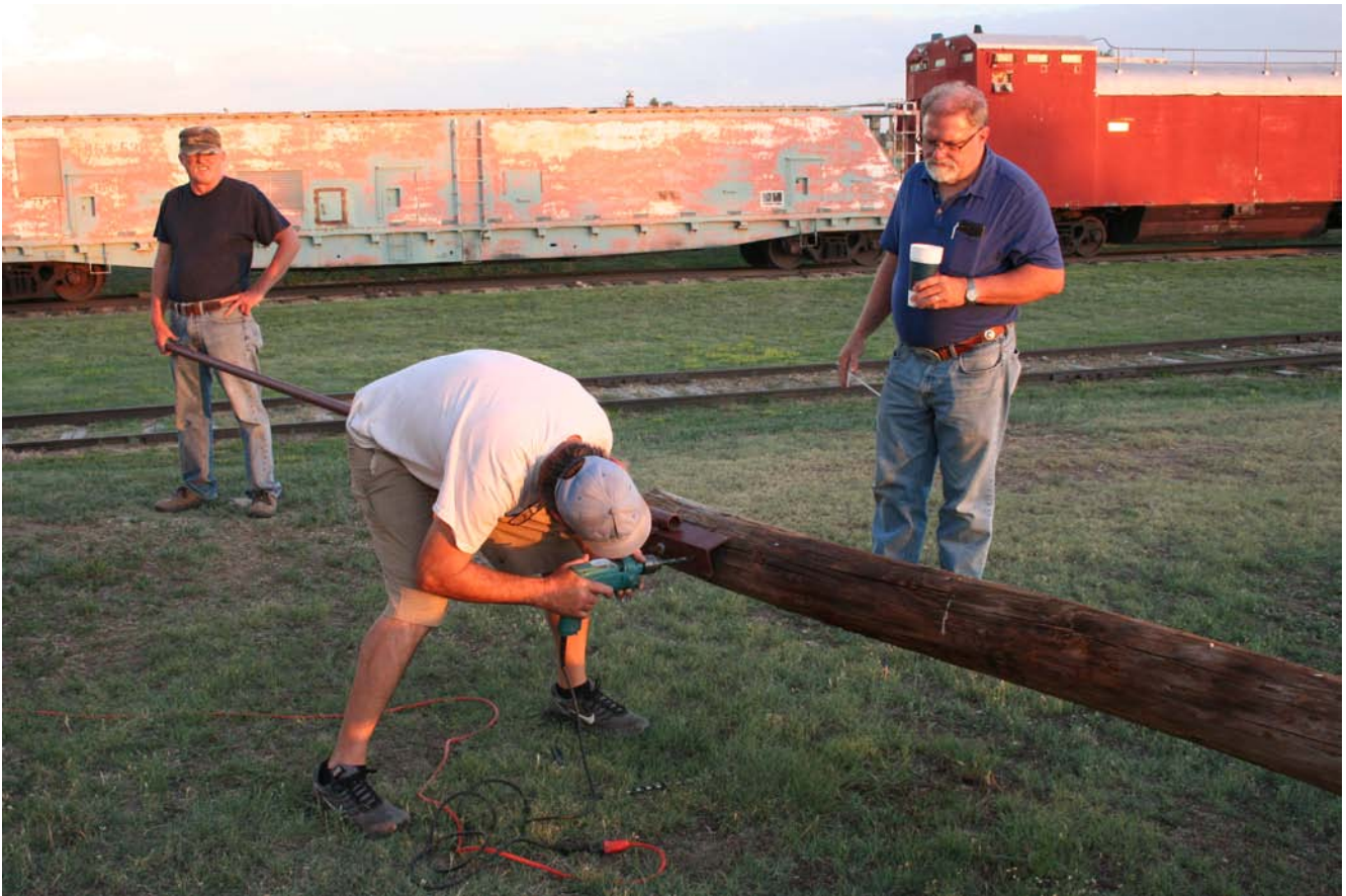
July 9, 2020: Above: Tracy had fabricated a 10-foot long mast as an extension to the utility pole and is drilling a pilot hole in the top of the pole to mount the mast while Chris holds the end of the mast steady and Kenneth observes the work. Below: The kit switch that had been abandoned behind Elementis had been moved onto ARM property.
