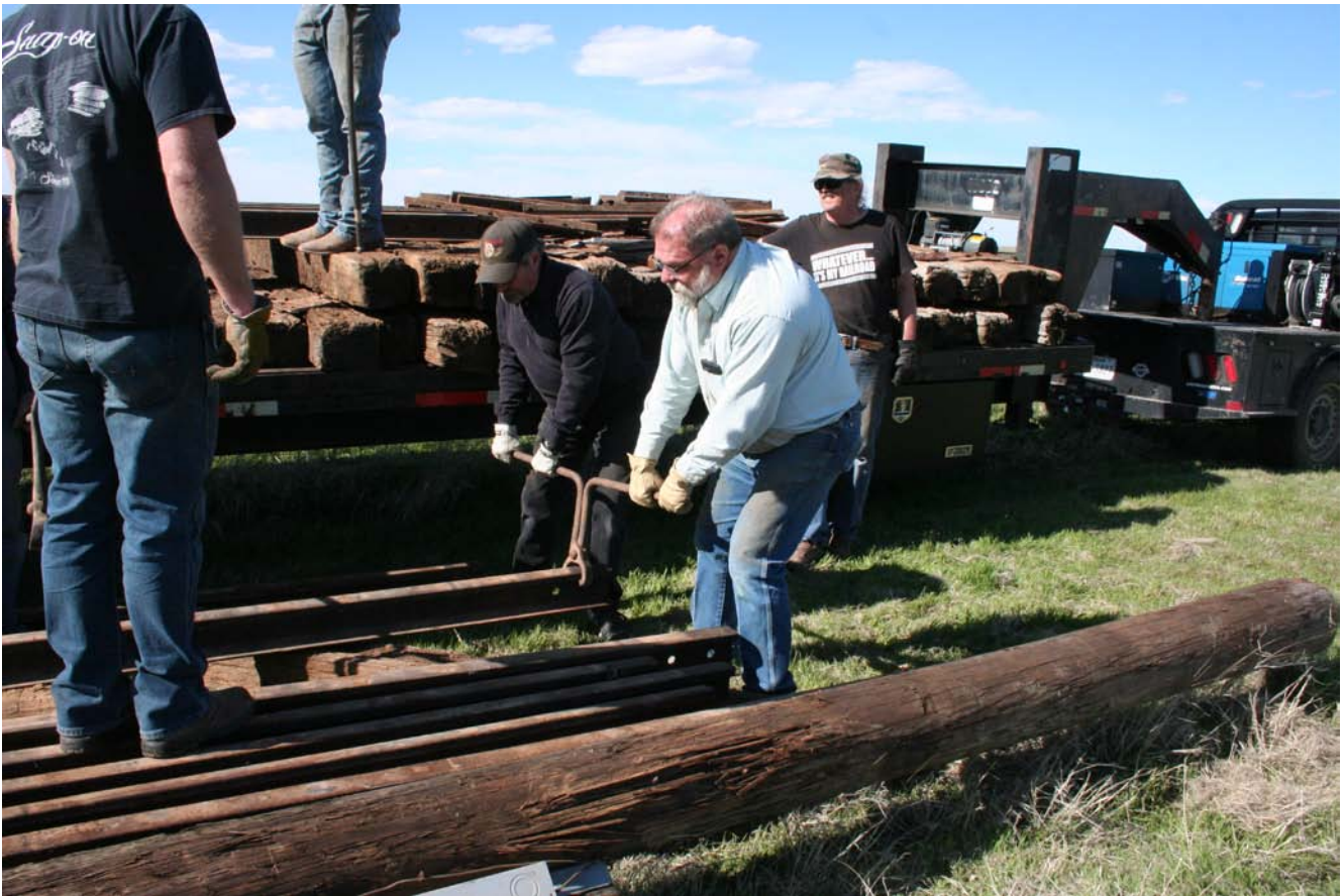
Above: The tools that Tracy fetched included a rail turner, rail tongs and tie tongs. This allowed the unloading to go much quicker with significantly less effort. Matthew is on the trailer rolling a rail toward the edge of the trailer while Bruce is attempting to help keep the near end straight, Chris is at the far end and Kenneth is standing out of the way.
