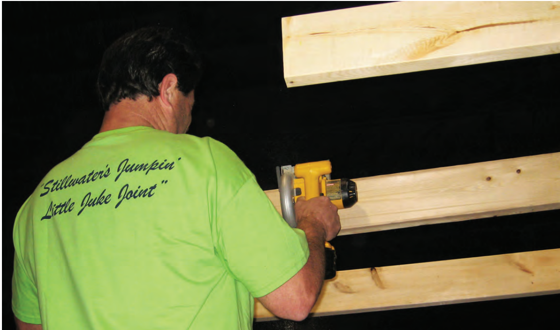
Carter Osborne cuts a joist to length.
