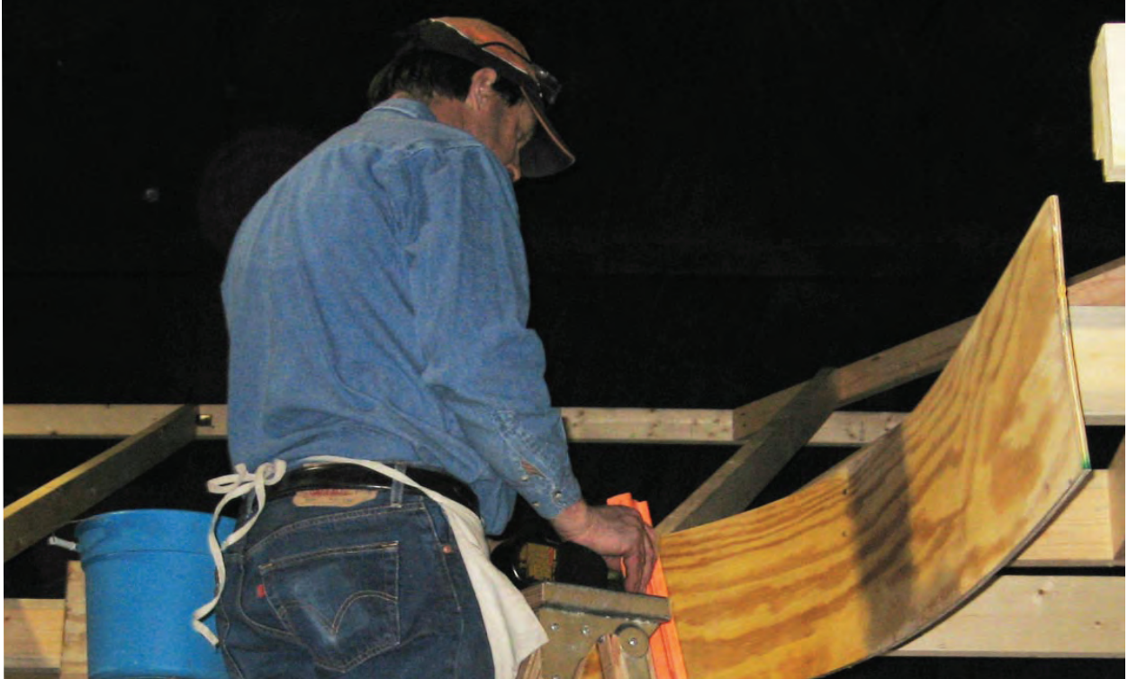
Tracy fastening his bent fascia after all rafters were installed. 2-19-09.
