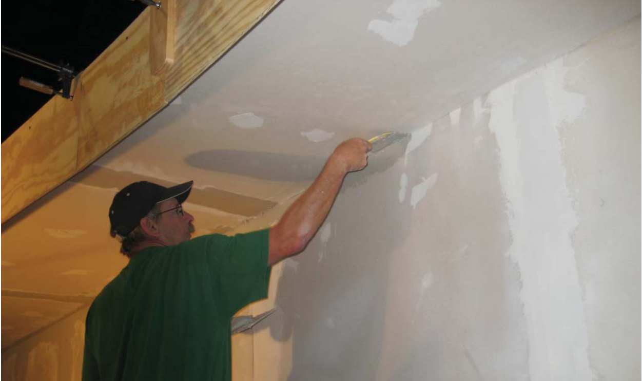
Earl Carrell taping and bedding the corner between the ceiling and backdrop near the south end of the layout.
