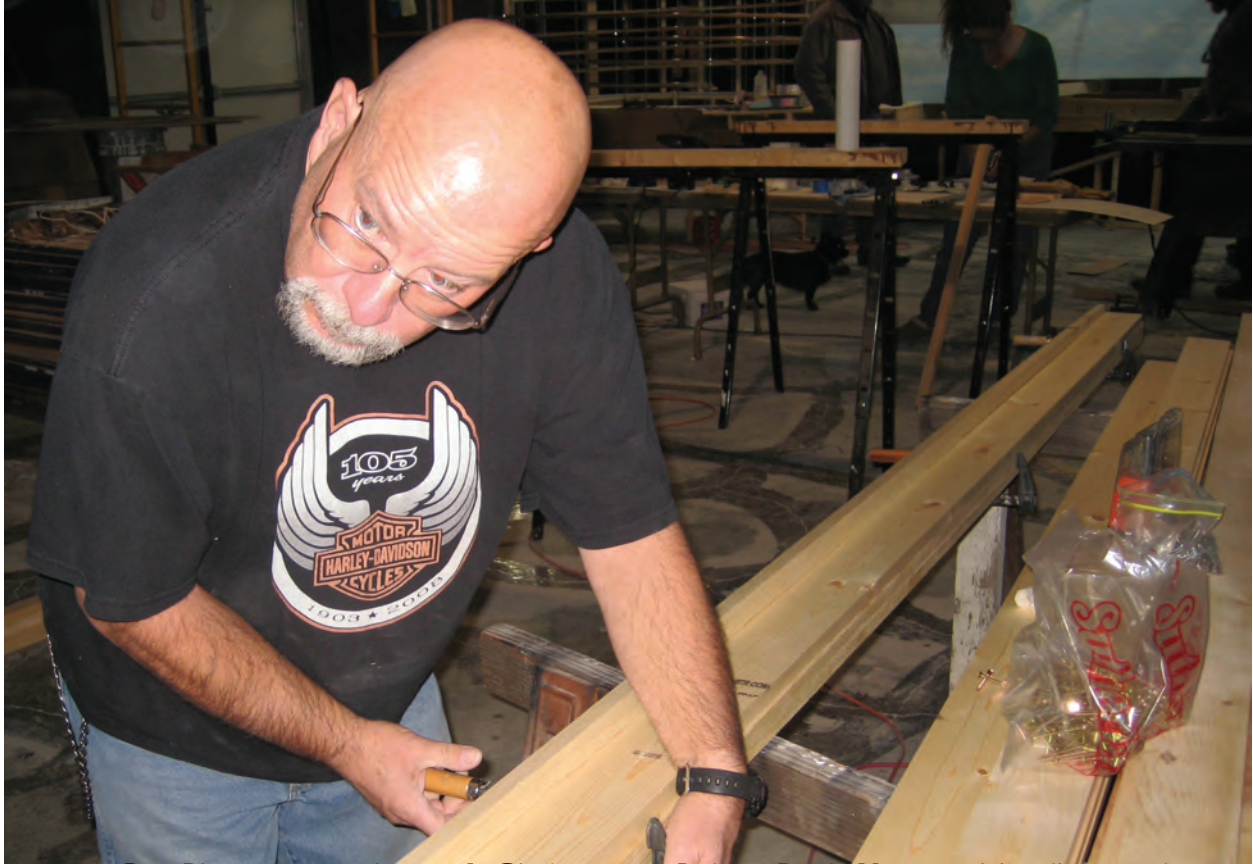
Above: Guy Pigg constructing an L-Girder
