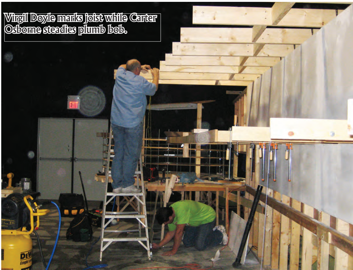
Virgil Doyle positions a joist using a brace to obtain correct spacing.
