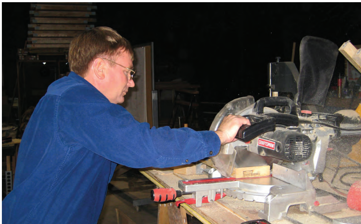
Bob Roth cuts a brace to length. It will go between the joists.
