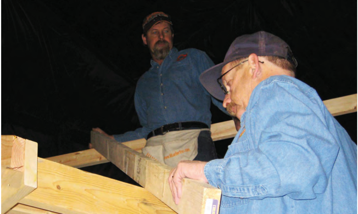
Tracy and Earl fit rafter in corner on 2-19-09
