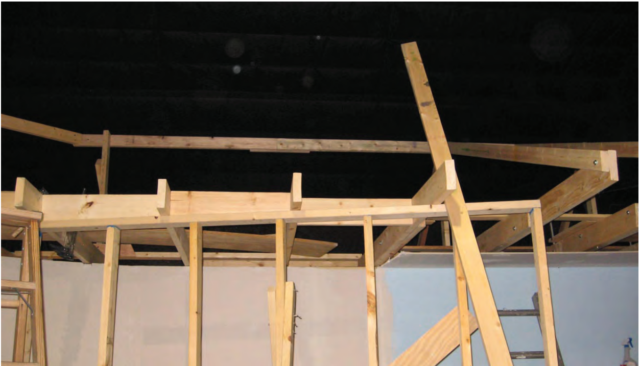
The South wall before the installation of rafters on 2-19-09
