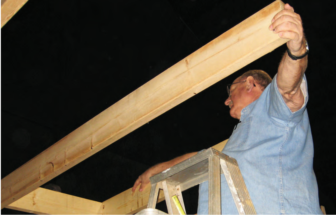
Virgil Doyle positions a joist using a brace to obtain correct spacing.
