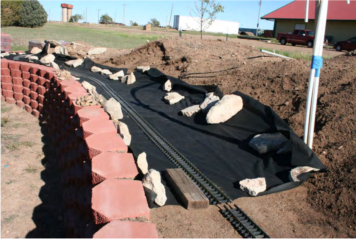
Garden: Weedblock fabric laid on the leveled track bed and sections of track laid in position.
