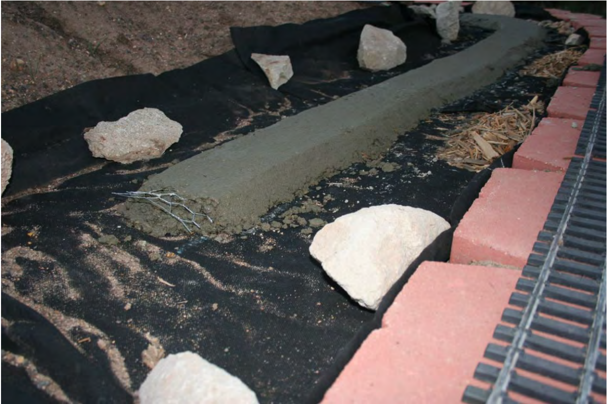
Garden: Weedblock fabric laid on the leveled track bed and sections of track laid in position.
