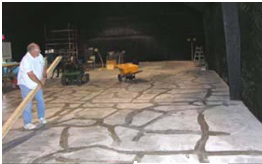
Treasurer Doyle drags out the first plates to build the new wall
