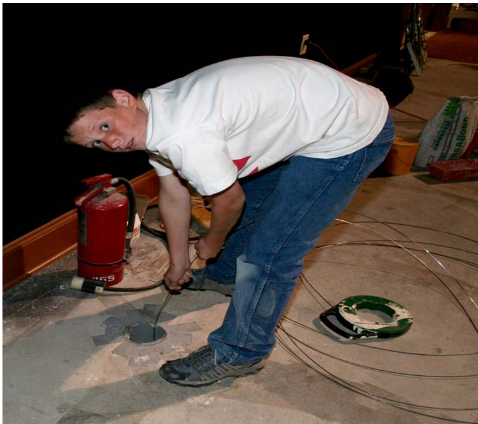
Adam Jones pulling electrical wire through floor conduit
