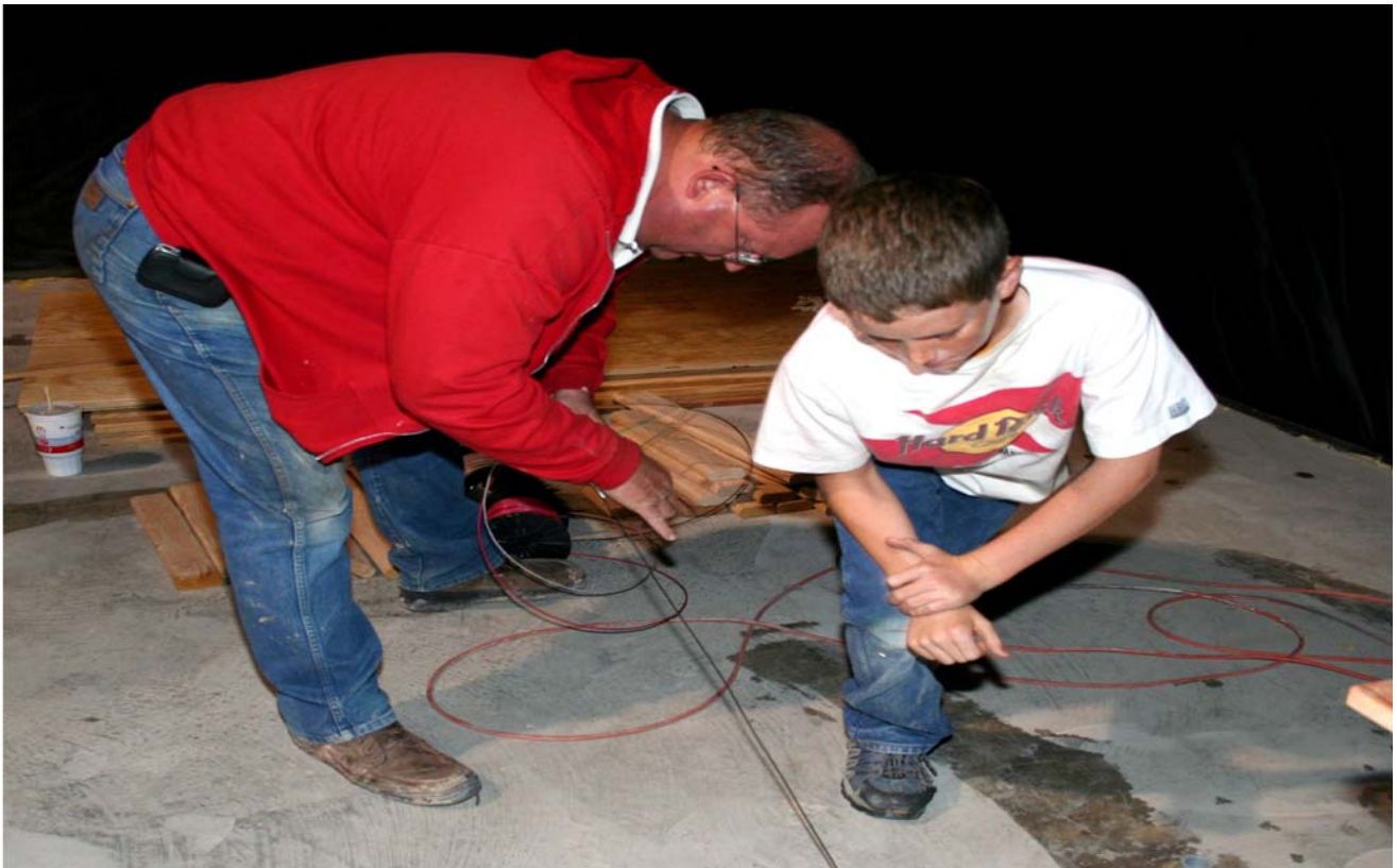
Tom Jones and Adam Jones prepare to thread electrical wire through floor conduit
