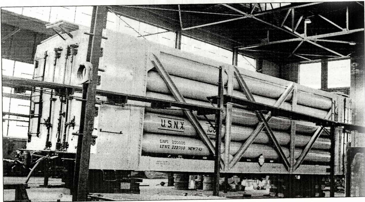
Third Generation: 30-Tube Car Built by GATC; November 1942 - August 1943 1013-1078
