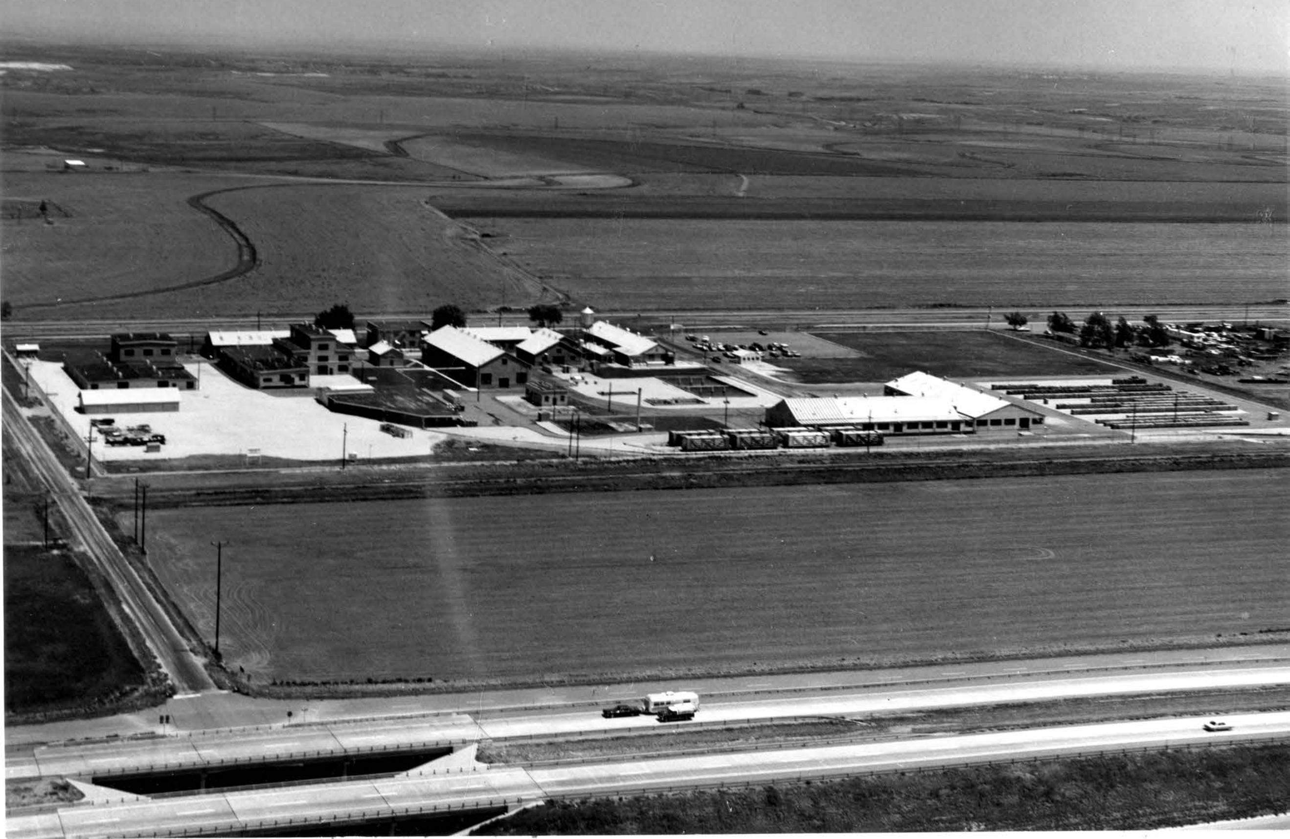
Amarillo Helium Plant 1980s looking north. I-40 is in the foreground.
