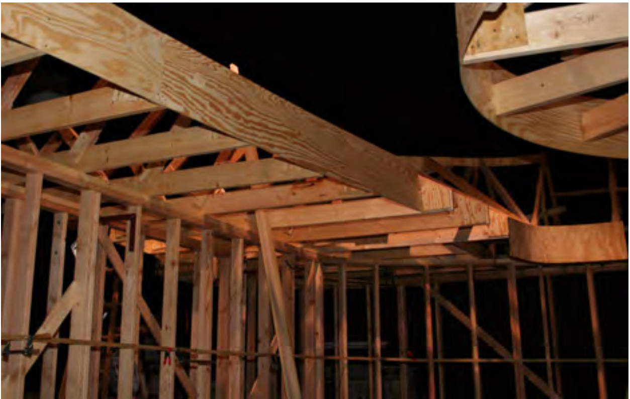
Inside West wall toward North end.
