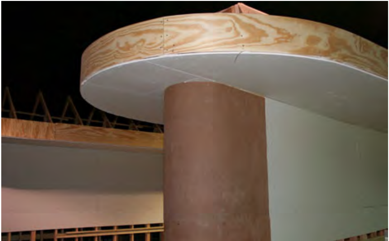
Composite material used on sharply-curved surfaces rather than sheet rock
