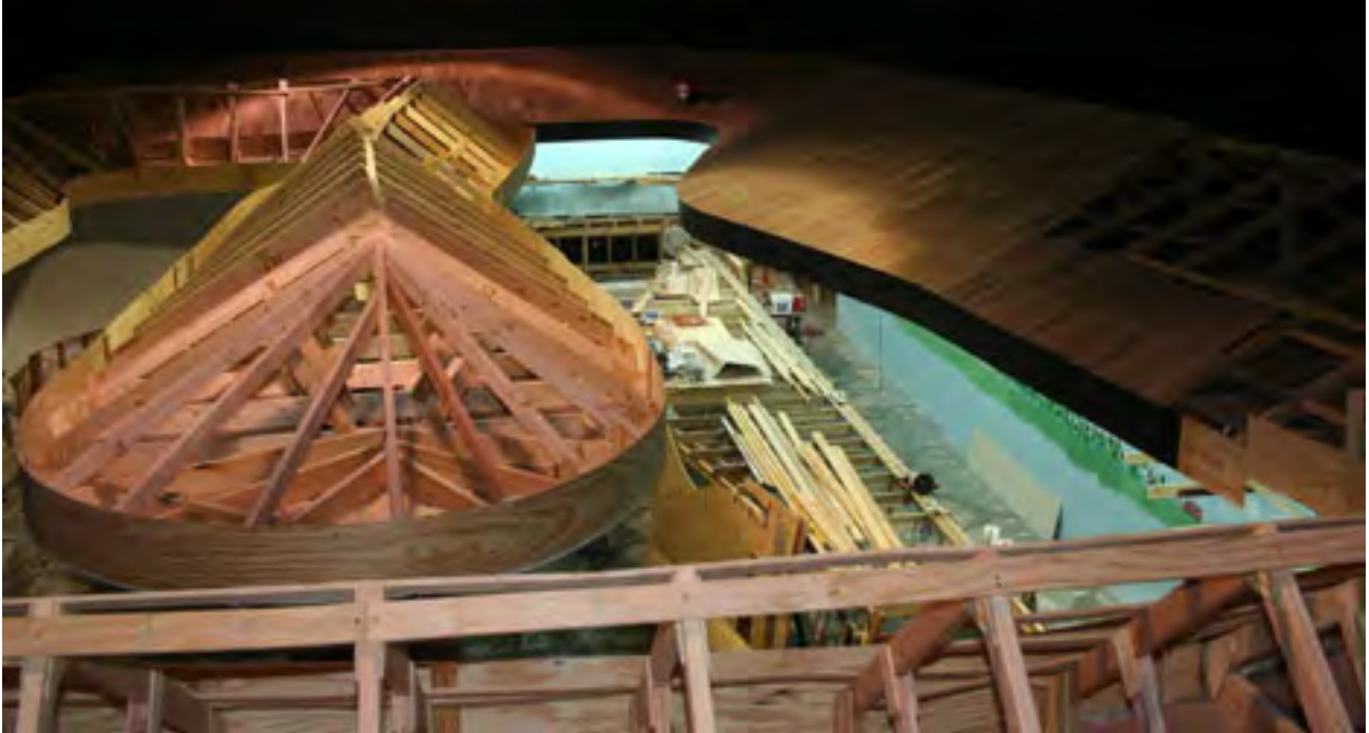
The south section of the roof and sheet-rocked walls.
