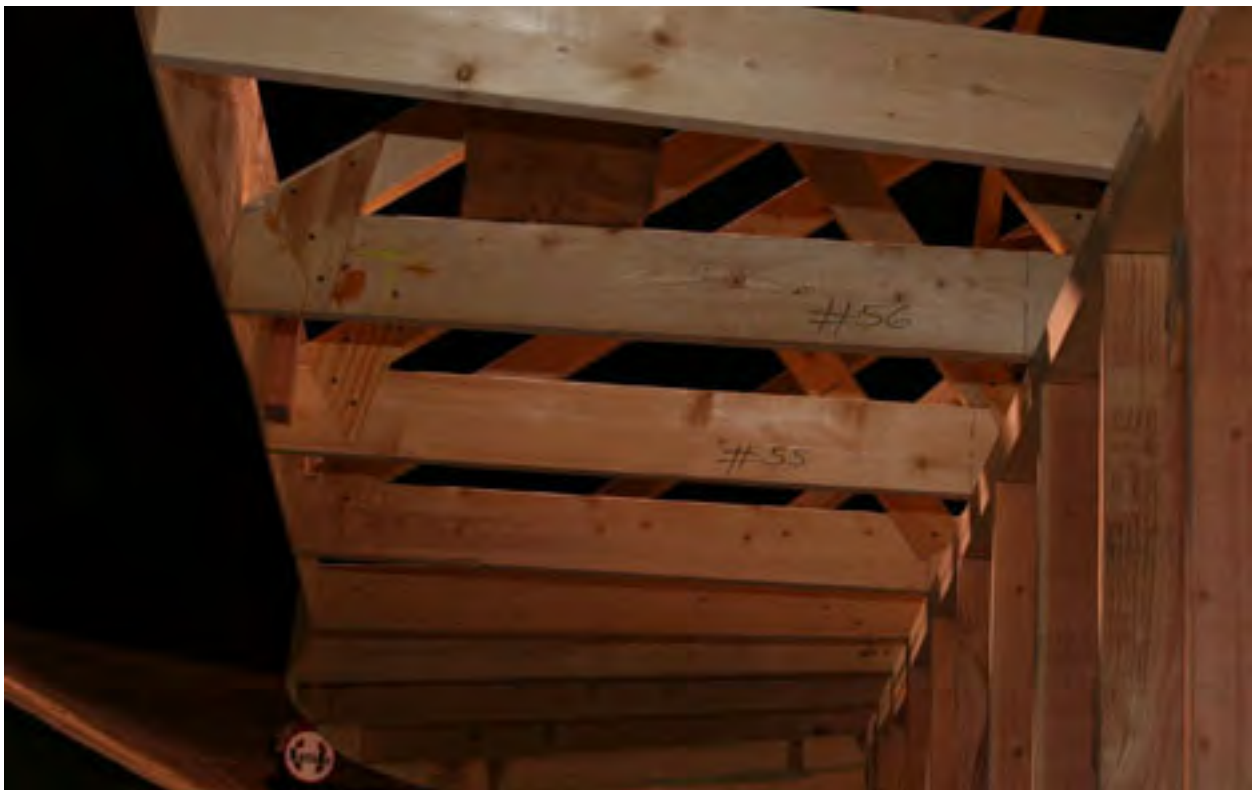
The East side of the big loop looking South.
