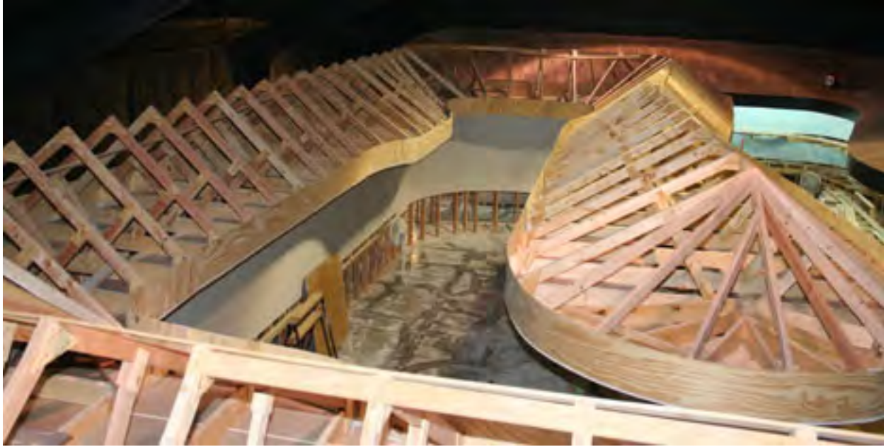
The north section of the roo and sheet-rocked walls below.
