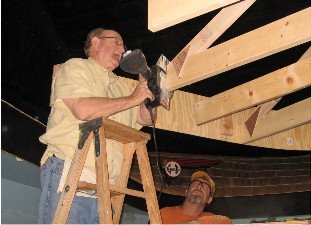
Virgil Doyle planing the ends of a girder.
