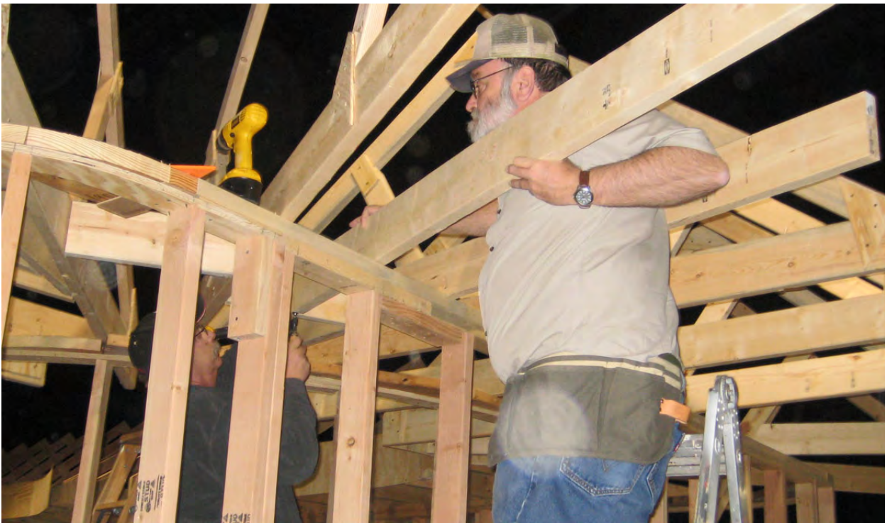
Jerry and Earl measuring length of joist.
