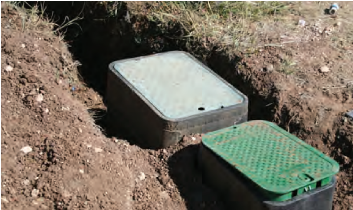
Two valve control boxes hold the cut-off valves and anti-backfeed valve that are connected to the water meter located just to the right of these boxes.
