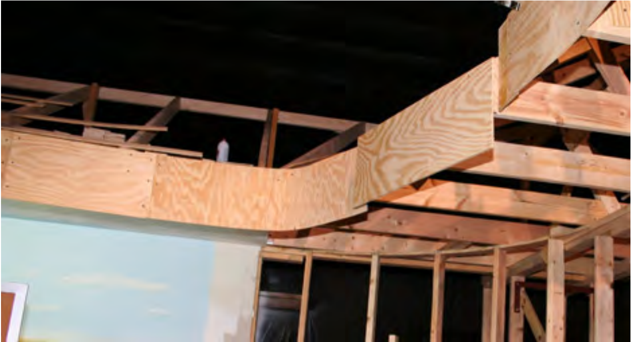
Inside West wall toward South end.
