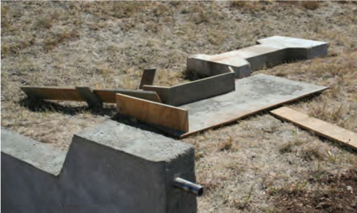
The surviving leg in foreground and the cast copy and form in the background. The pins on the end enter holes in the bottom of the electrical cabinet. Threaded internally.
