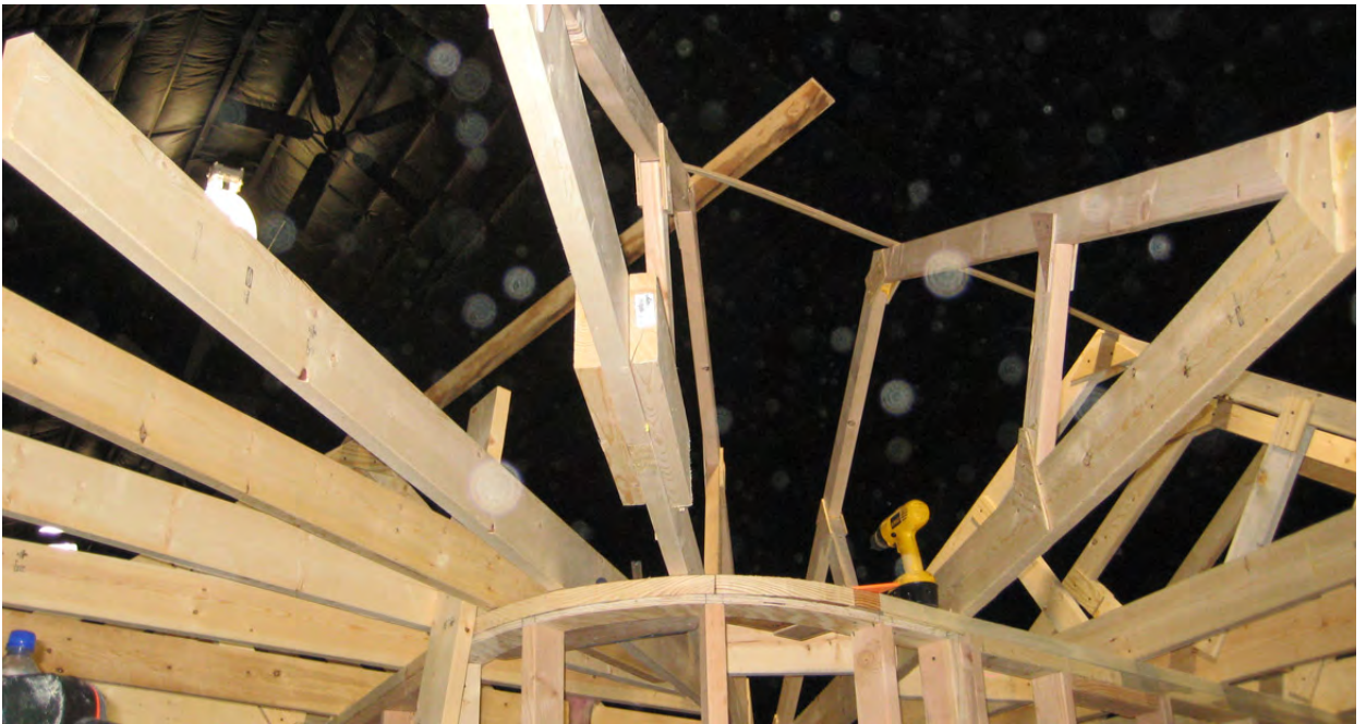
Southeast corner partially completed.
