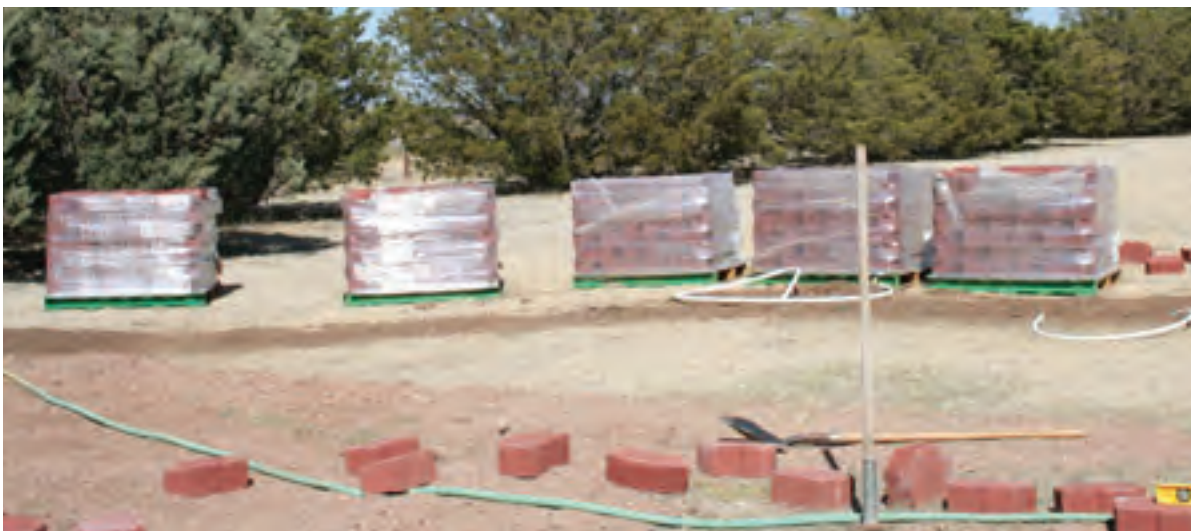
Tracy moved all of the pallets of stone on Friday September 30.
