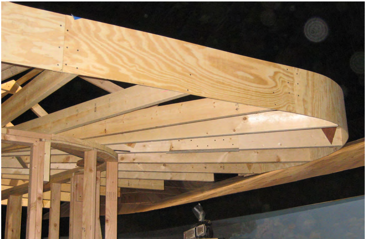
The Big Bend from the back side. The first piece uses the long grain cut of plywood. The joint on the right end begins using plywood cut across the grain which allows the sharp bends with little wetting. When covered with black formica, it will be difficult to tell the difference.
