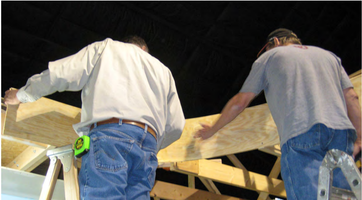
Jerry and Earl make first attempt at bending fascia by wetting the long grain of plywood.
