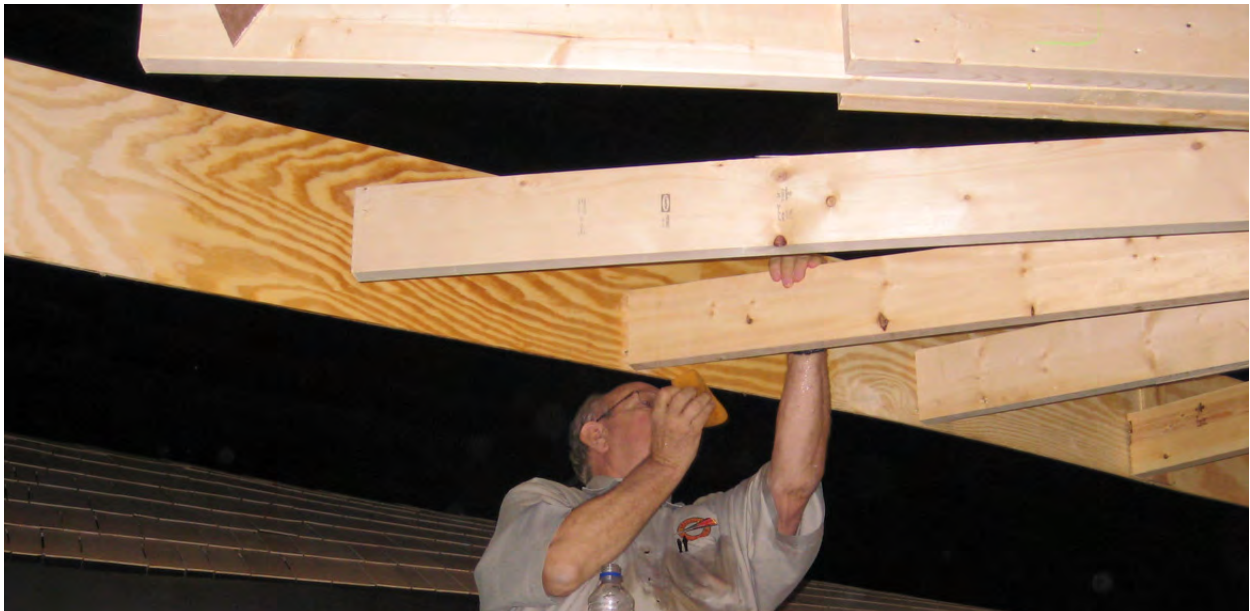
Virgil Doyle makes first attempt at the Big Bend by wetting the long grain of plywood.
