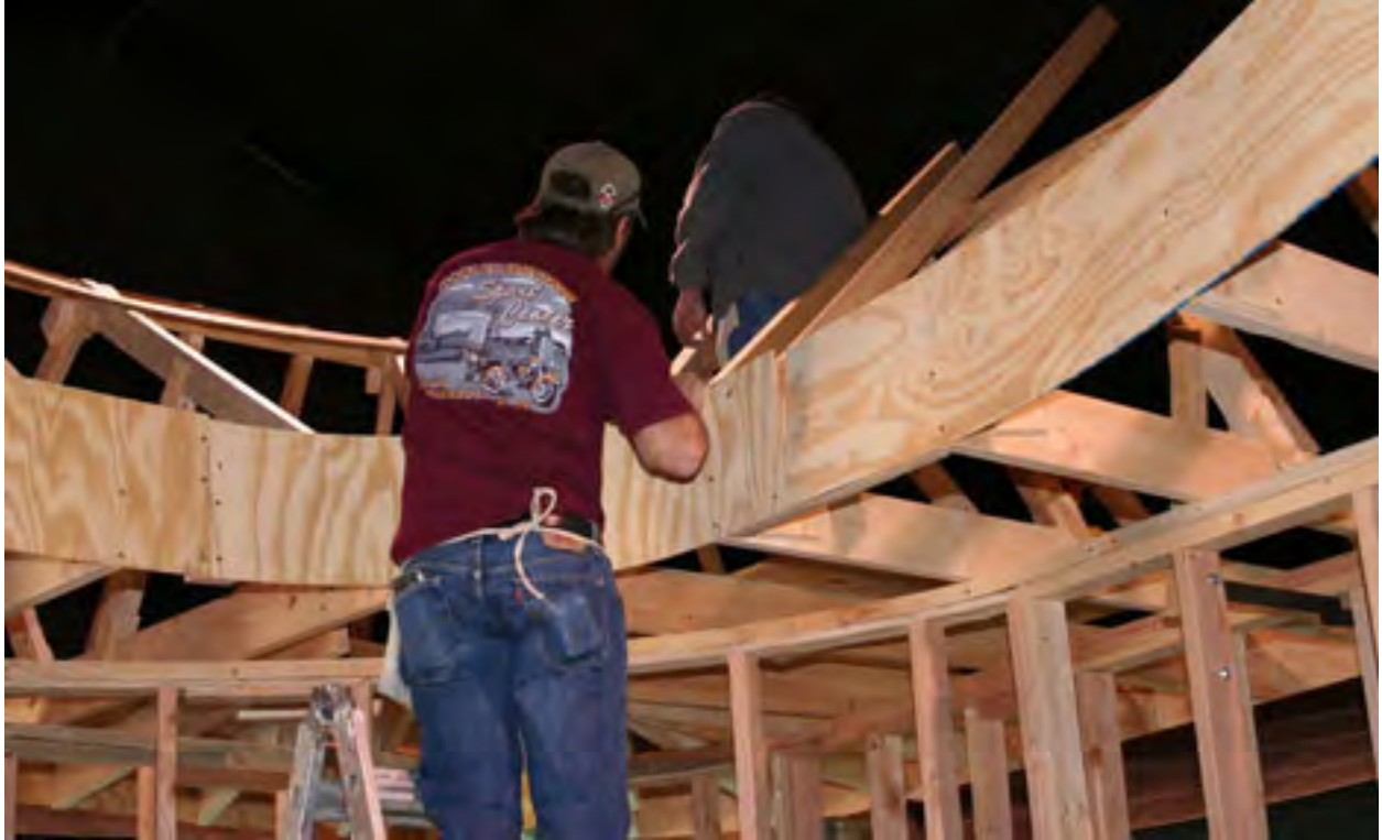
Tracy Ball and Earl Carrell are adding SE corner rafters.
