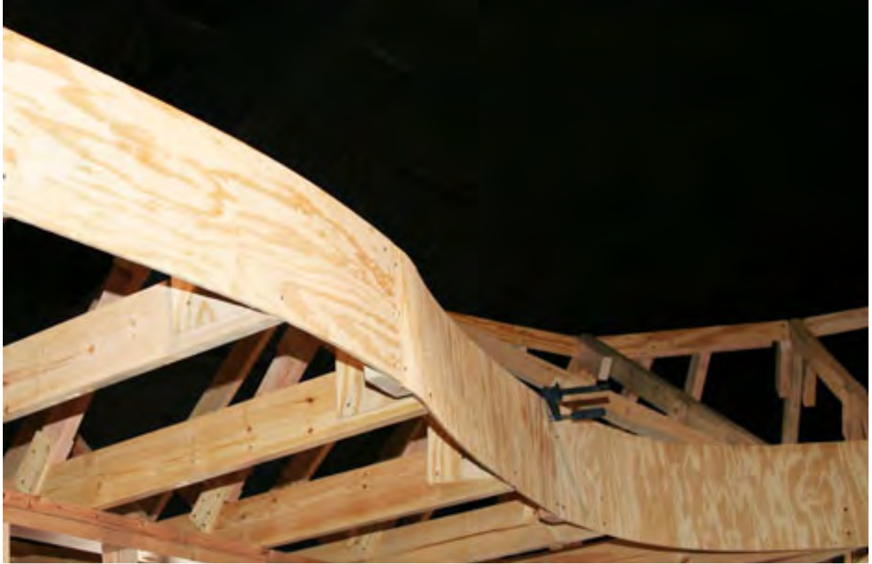
The complex curve that Bob was working on after closure. The clamp detracts from the flow.
