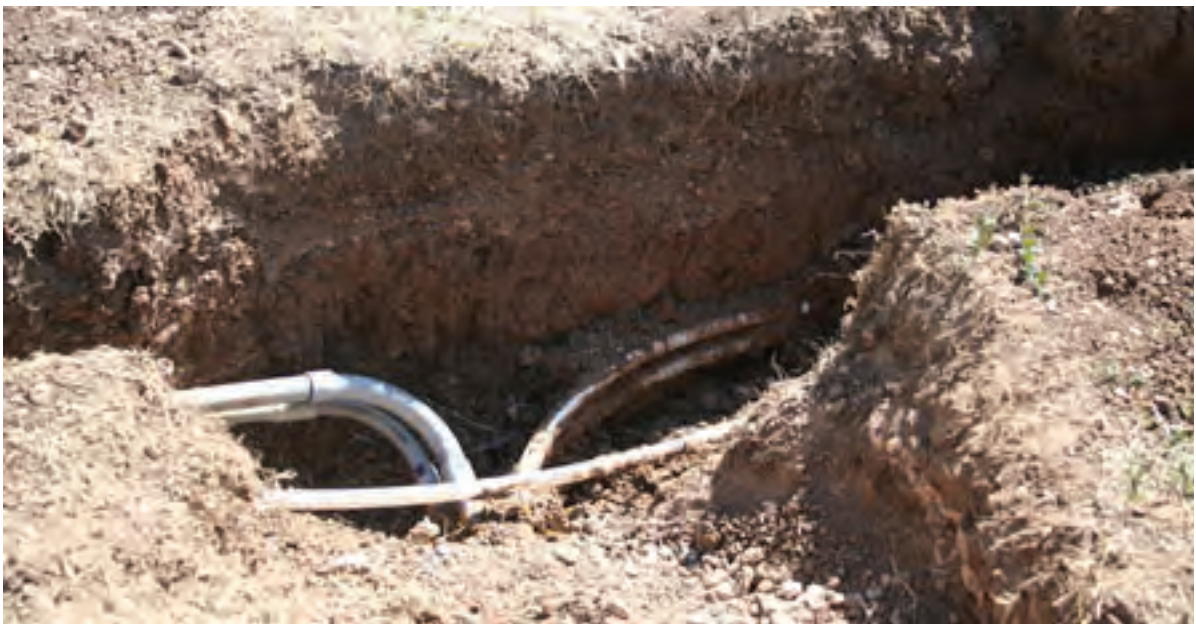
Ditch for Timer control wires.
