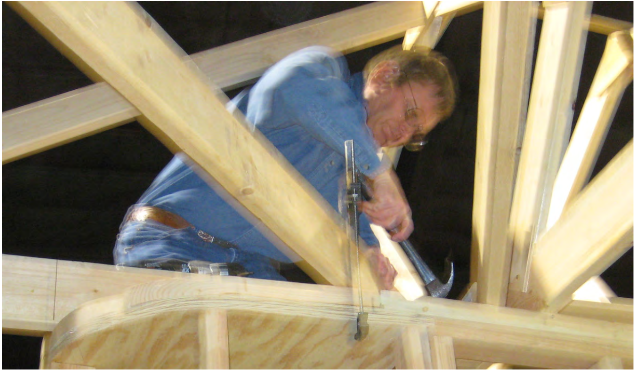
Bob Roth working on girders at end of peninsula.
