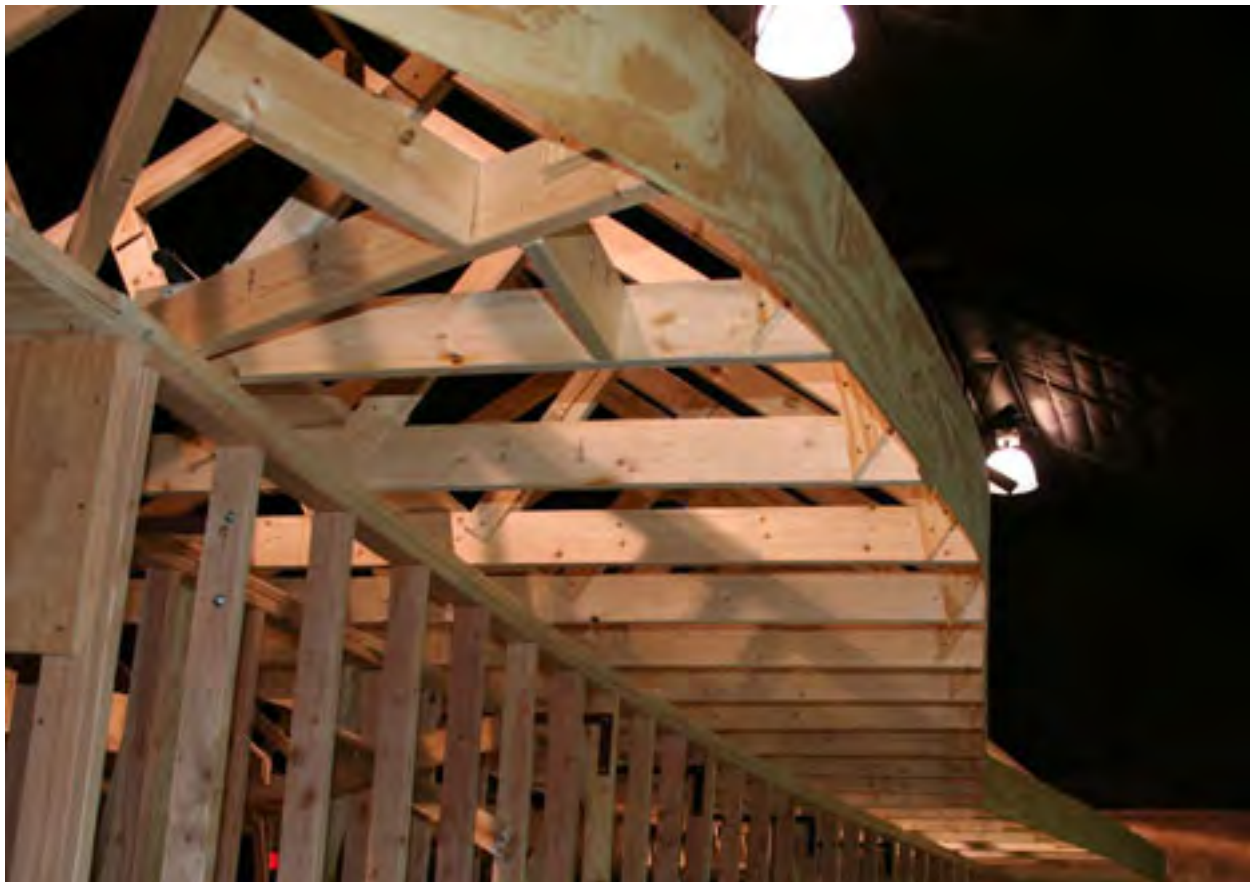
Fascia installed along the South side of the peninsula.
