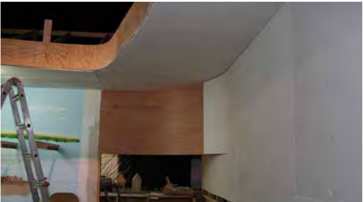
The southwest inside corner.
