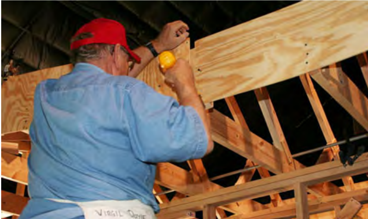
Virgil Doyle is closing the gap at the SE inside corner.
