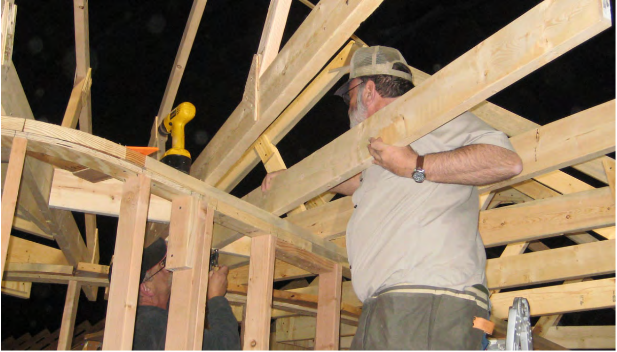
Jerry and Earl fastening joist in place.
