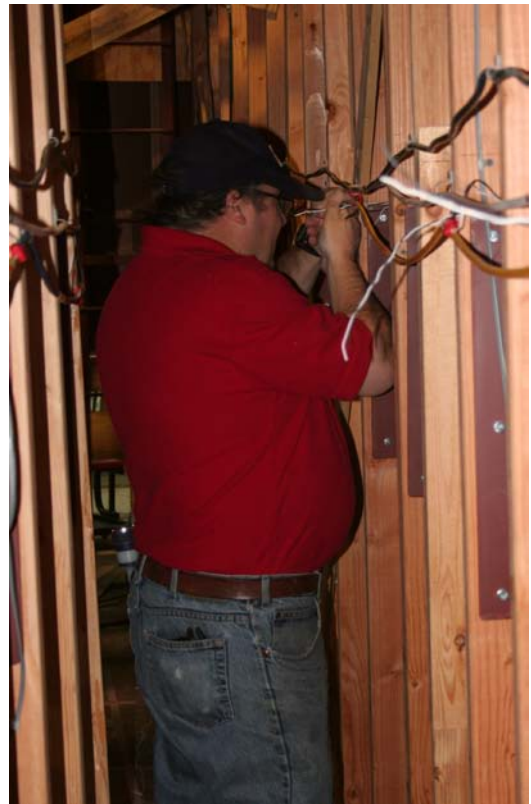
December 14: Left: Bruce Carter twisting wires for one of the power drops from the track while Rhett looks-on, standing ready to hand some tape to Bruce. Right: Jimmy Snavelly behind the wall pulling the wires thru after Bruce twisted them together and tied the ends with a piece of tape.
