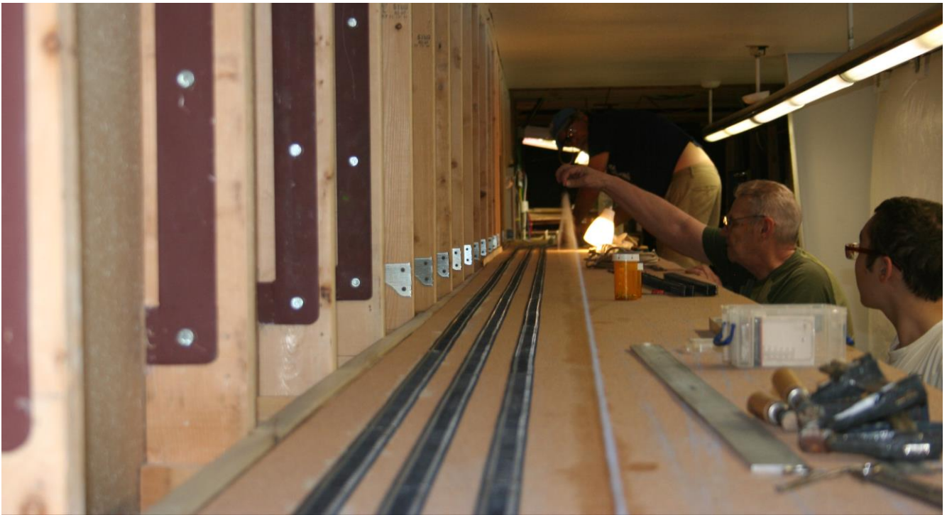
June 7, 2018: Upper Staging Yard – Floyd preparing to snap a chalk line for one of the tracks; Tracy is holding the far end of the line while Gabe looks on.
