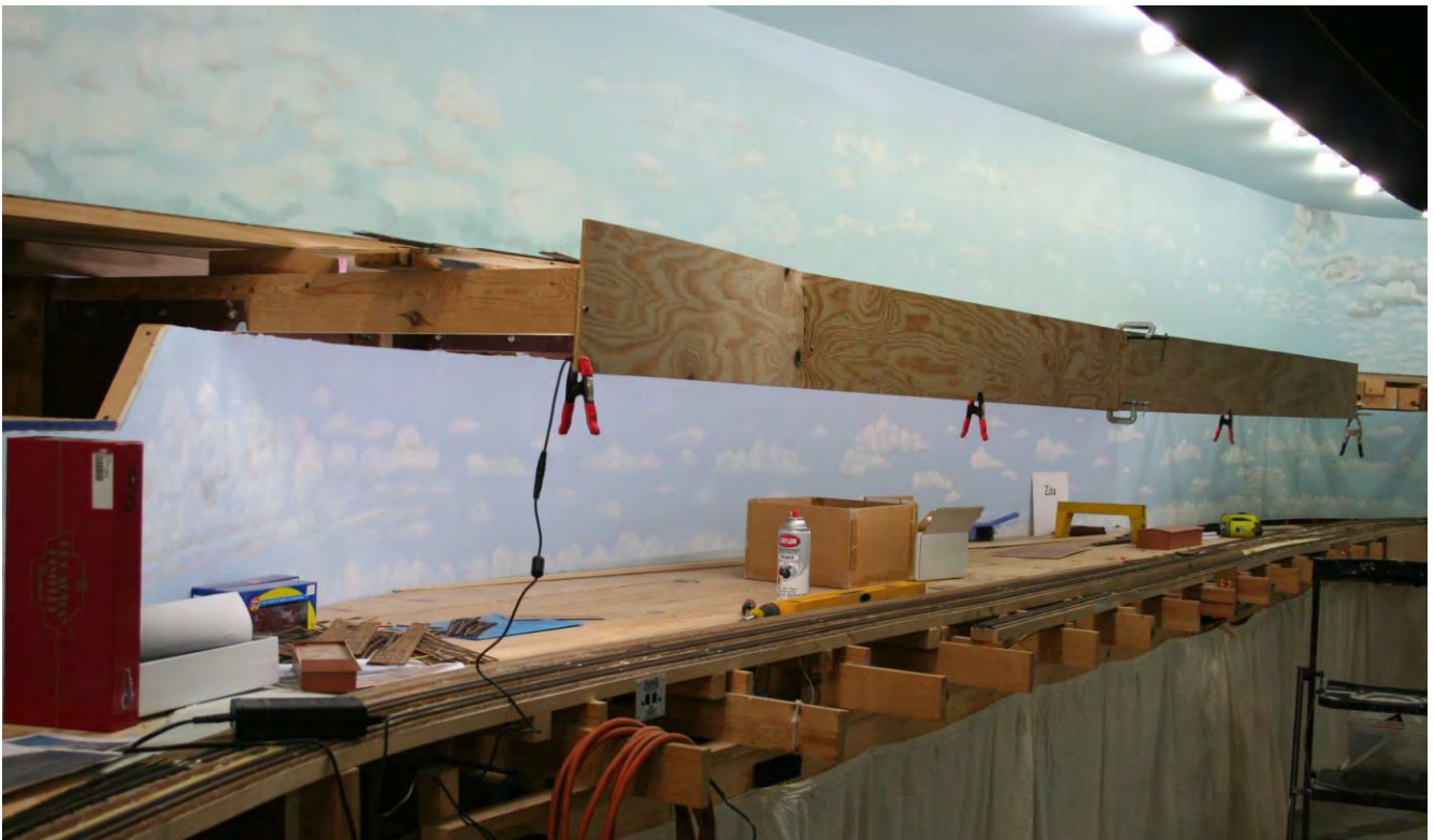
February 27: LED lighting strip now clamped to fascia piece temporarily secured along the edge of the upper level. There is a noticeable color difference between the two levels despite the fact the blue color on the backdrop wall is the same color.
