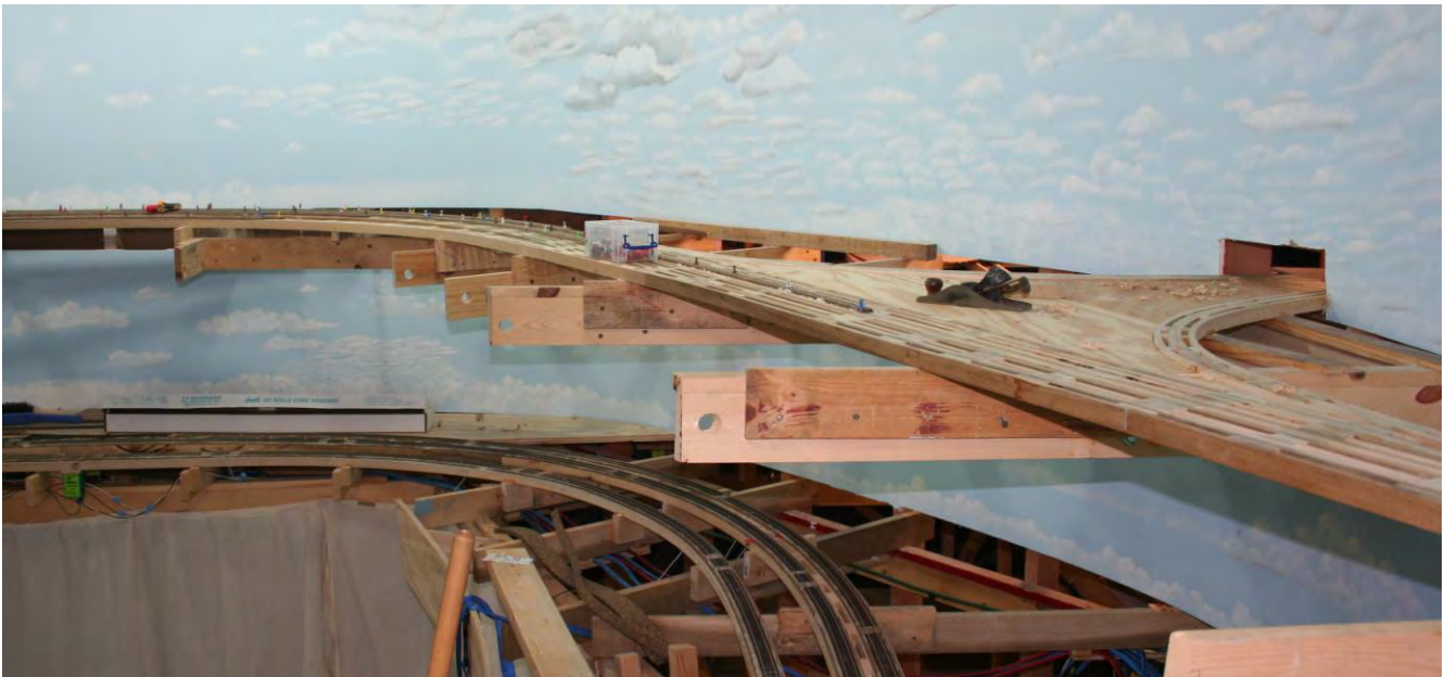
The completed spline roadbed for the wye for Lubbock Junction in Canyon on the second level of the layout. Note that plywood decking was installed between the legs of the wye.
