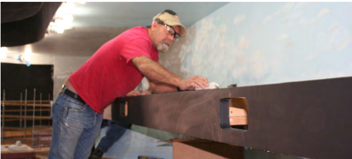
April 26: Tracy Ball sanding cork roadbed on upper level in Canyon. Behind Tracy, Guy Pigg is working to install a turn-out.
