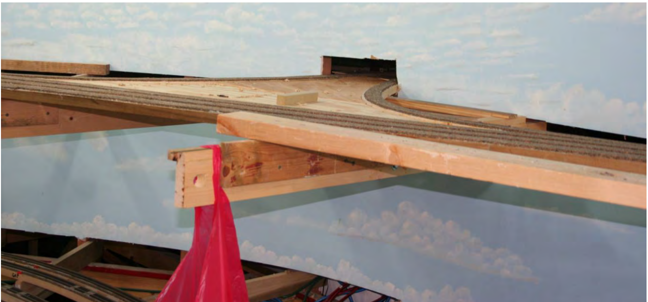
February 22: Cork laid on the Lubbock Junction wye at Canyon is now ready for track.
