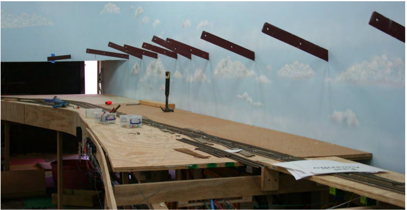
Aug. 23: Vicinity of East Tower: Upper level support braces inserted thru the slots in the wall so a count could be made to determine how many more are required.
