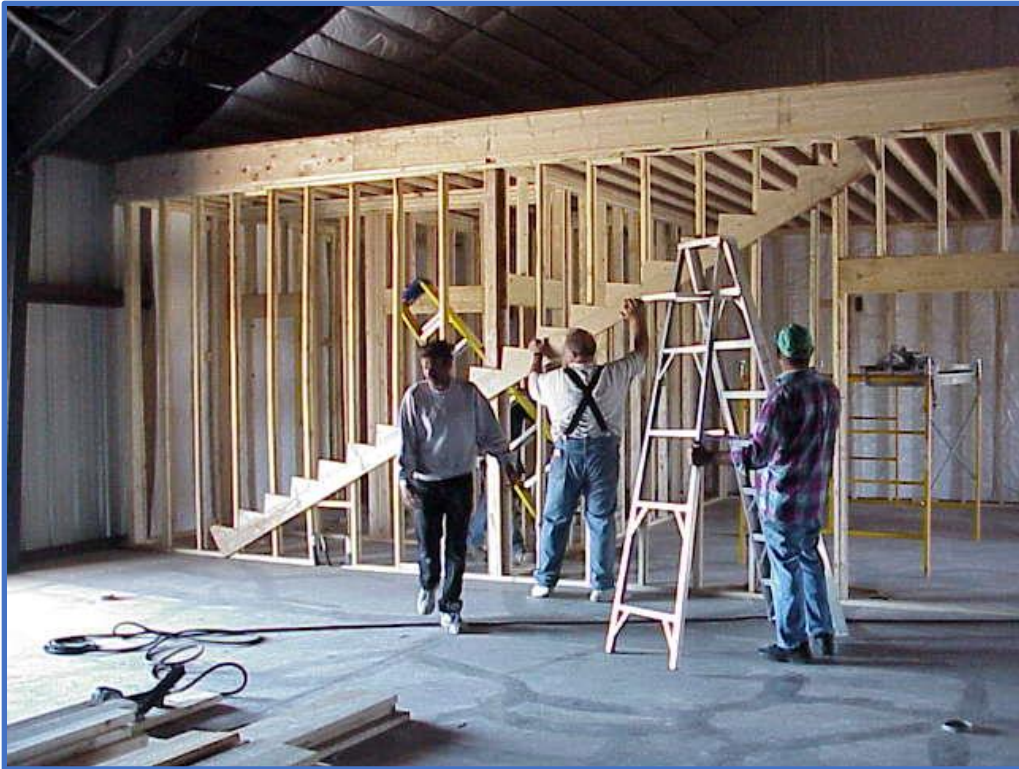
Top. Interior framing went rather quickly if we had a good supply of wood and nails. Tracy Ball, Tom Jones, and Earl Carrell are hard at work installing the stairs to the loft. Bottom. A view of the rafter structure in what became the interior ceiling of the layout.
