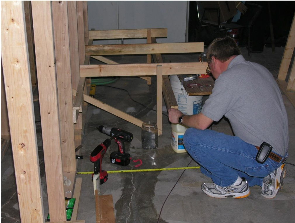
Top. A final look at the framing finds Bob Roth measuring before installing lower-level framework. Note the L-girder on the left. Bottom. A very happy crew. Left to right; Tracy Ball, Bob Roth, David Jusiak, Virgil Doyle, Guy Pigg, and Jerry Michels stand amid the center peninsula framing. Soon drywall installation begins. We hired a local craftsman to make sure the tight curve at the end of the peninsula was professionally done.
