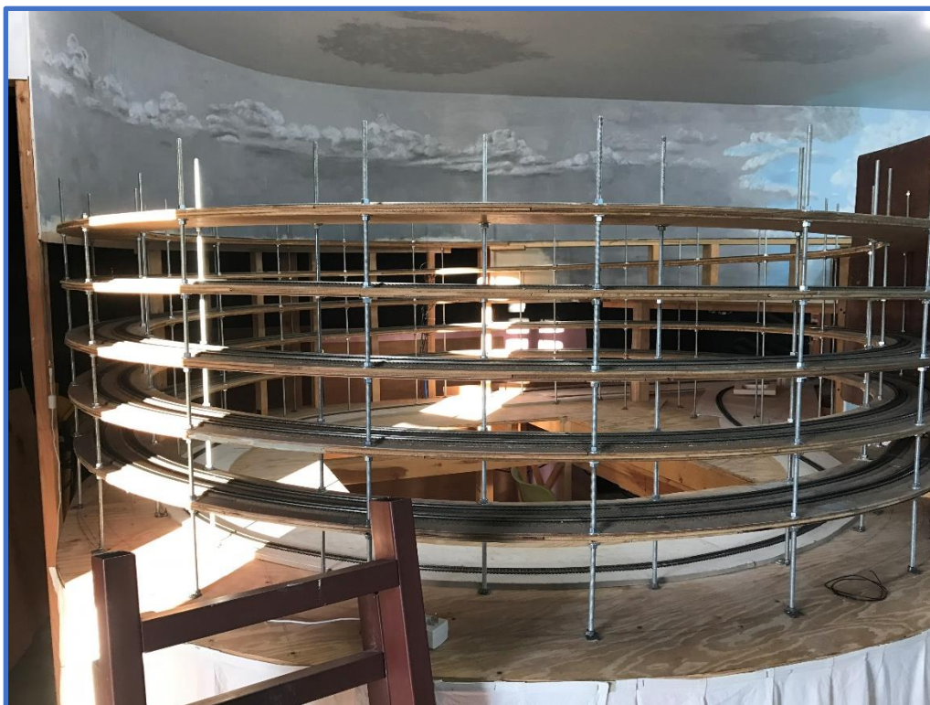
Top. A key component of the layout is connecting the lower to the upper level. Tracy Ball built an innovative double-tracked helix with threaded rod and nuts to adjust the rise of the sub-roadbed to a comfortable 1.3% grade. Bottom. A bit further down the road, is a photo of the helix in place.
