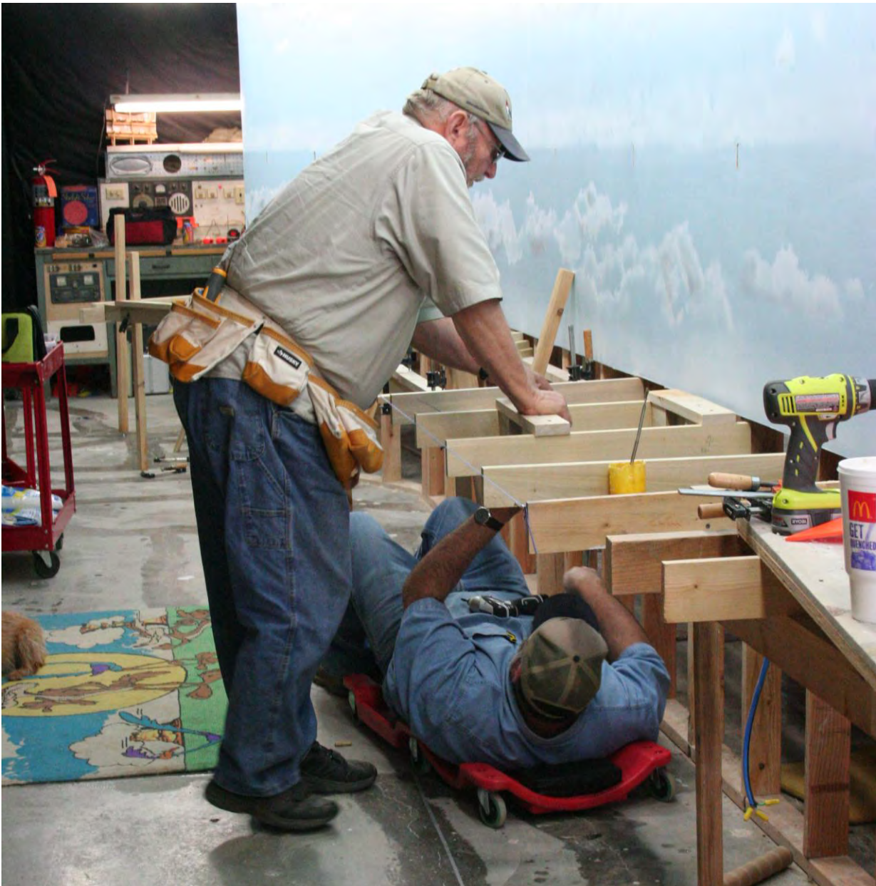
3/23/1013: Virgil Doyle and Jerry Michels working on installation of joists at Canadian after work on L-girder was halted.
