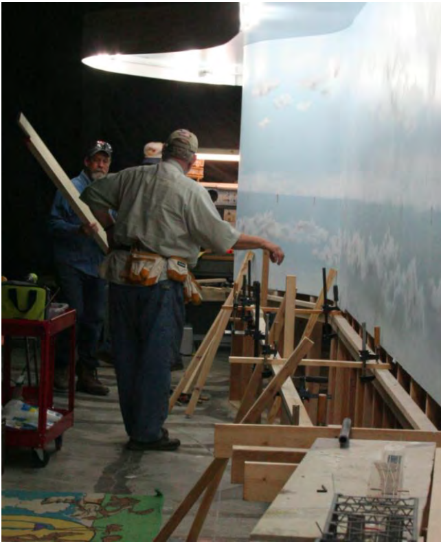
L-girder at Canadian is being extended toward the curve at the Northwest corner of the layout between Canadian and Miami. Work paused for a moment so Tracy Ball, Jerry Michels and Virgil Doyle could look toward the camera.
