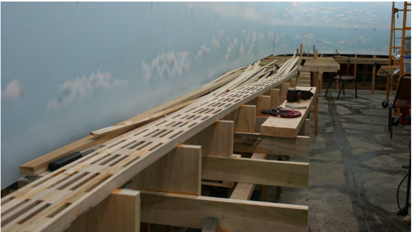
New spline roadbed extending toward the location of the City of Panhandle on the layout. Elevation of the spline is dropping.
