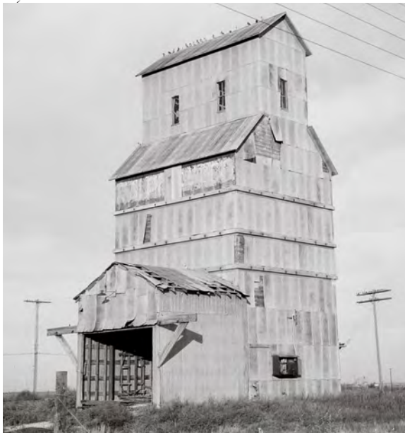
Ralph, Texas elevator on November 11, 1974. Southeast view left above and north-east view right above. The wooden framework is covered with corrugated iron.
