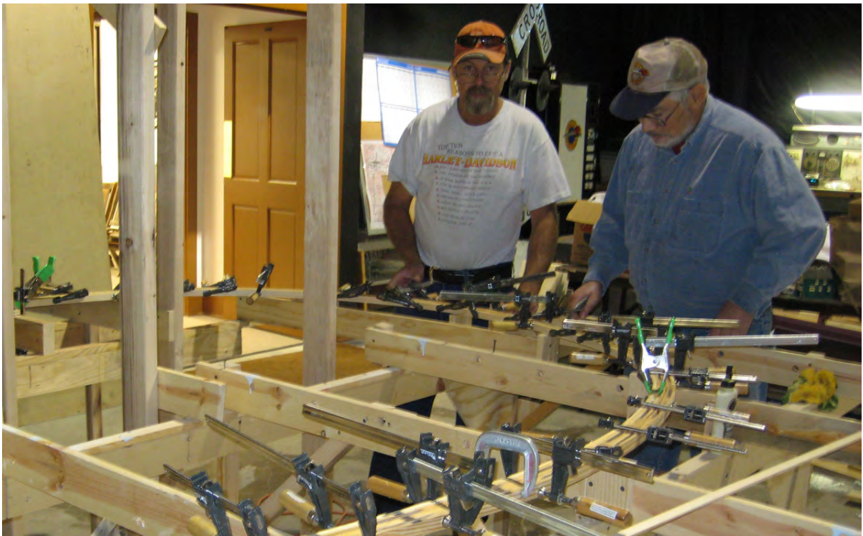
TRACY AND MIKE JONES CHECK OVER THE INSTALLATION.
