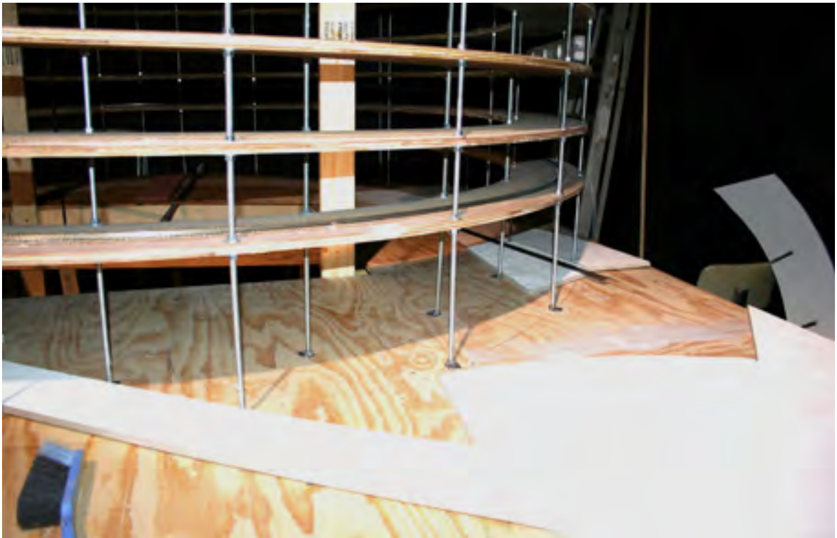
Homosote for the return loop has been placed inside the rods supporting the helix. Homosote is in the process of being placed for the tracks connecting the loop with the lower staging yard.
