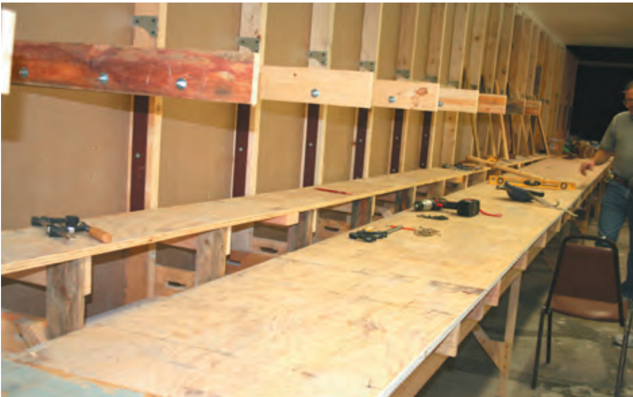
The Rock Island and Ft. Worth and Denver yards are approximately six and one-half inches above the lower level of the staging yard. This ten-inch wide ramp will allow trains from those yards to enter the staging yard lower level.
