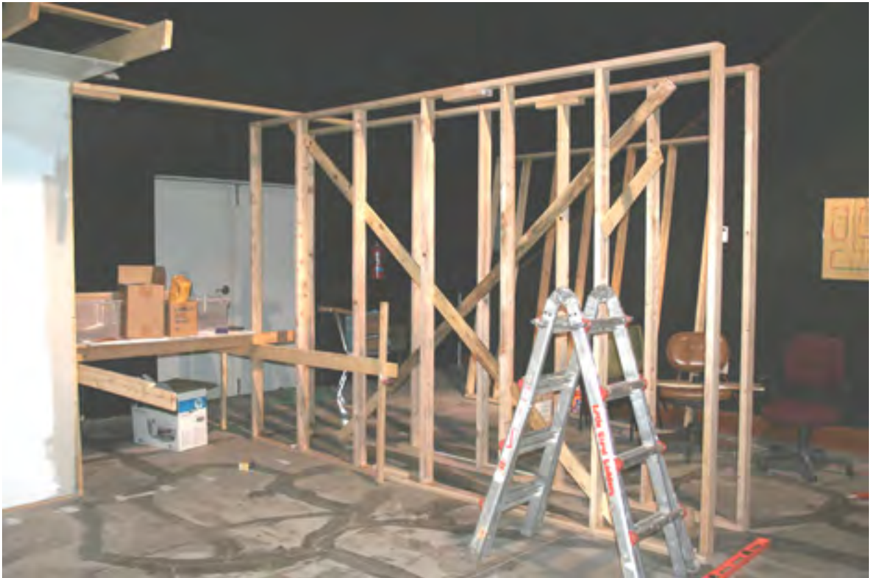
East side view of the new twin walls constructed Saturday, January 28. These two walls will support the temporary return loop bench work. Later they will support parts of the East Tower vicinity in the Amarillo yard on this side and the Canadian yards, including the wagon bridge and the railroad bridge on the west side. The upper level will support Umberger on this side and Texico, NM on the west side.
