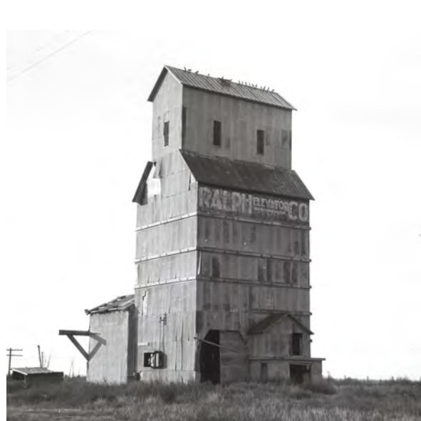
Ralph, Texas elevator on November 11, 1974. Southeast view left above and north-east view right above. The wooden framework is covered with corrugated iron.
