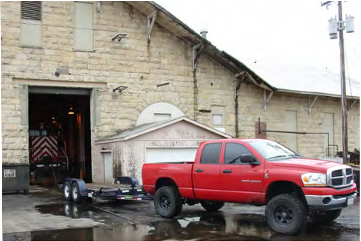
The Jacks have just been unloaded at the Nebraska Central Shops. It rained there also.
